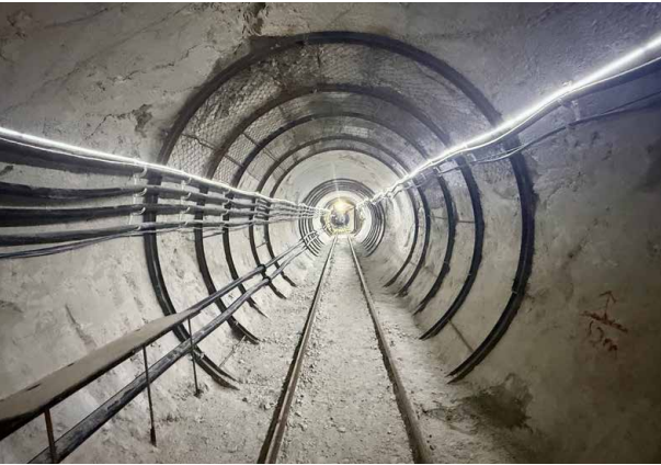
▲ 江铜银珠山项目巷道成型 Tunnel Formation at the Jiangxi Copper Yinzhusan Project
